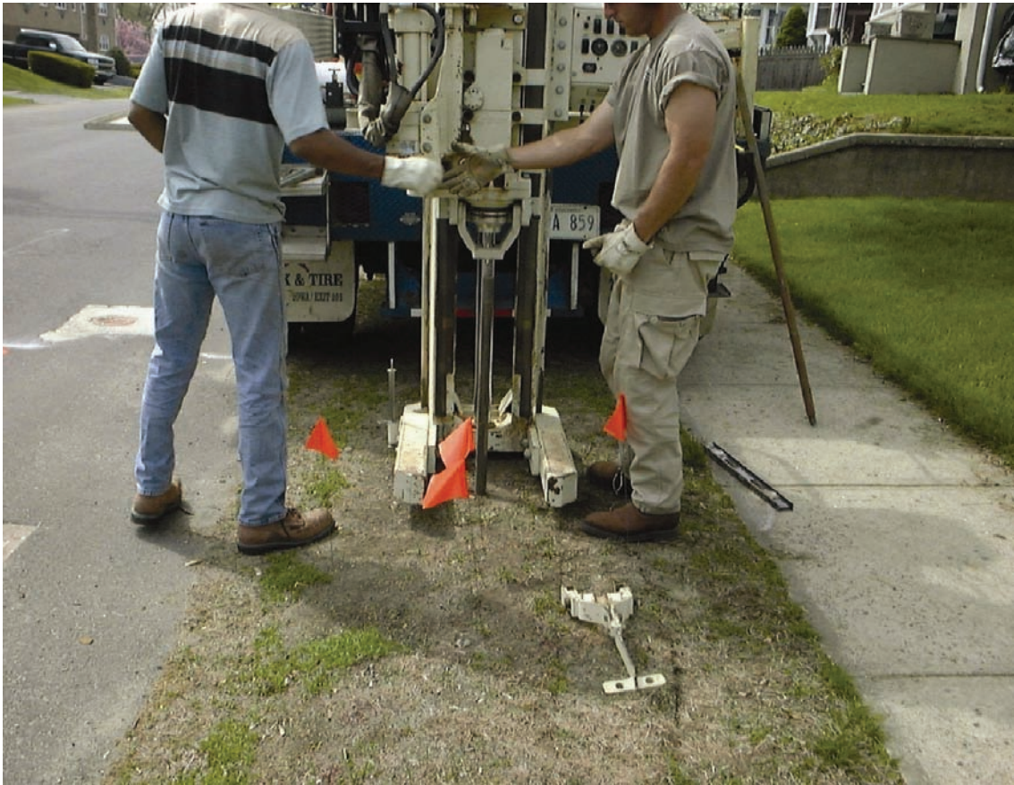
Figure 31. Photograph illustrating five PRT sample locations (orange flags) near MW213.
